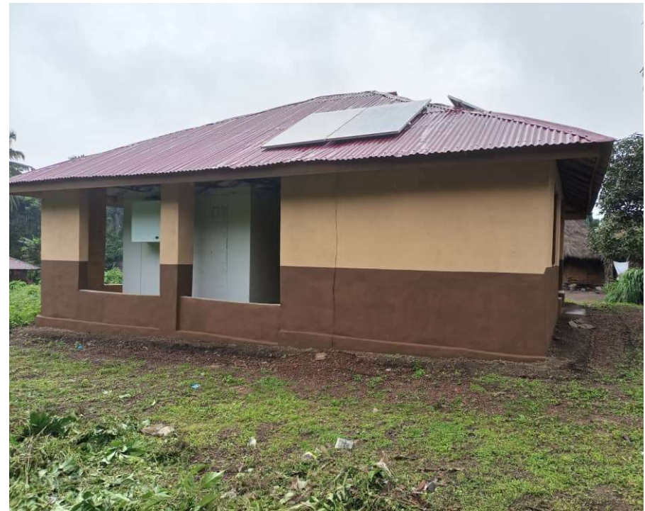
Solar-powered cold room facility in Najay village – the community contributed by building the cold room house
